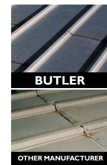
Other Manufacturer Above Top: Butler staggers panel splices to avoid the four-corner condition—another design feature to assure weathertightness and longer roof life. Above Bottom: Most manufacturers locate panel splices at exactly the same position across the roof. This four-corner condition is very difficult to seal and keep weathertight.
