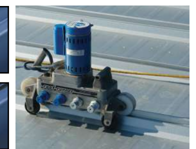
This seaming process uses a heavy-duty four-stand, electric, portable roll-forming machine called the Roof Runner.
