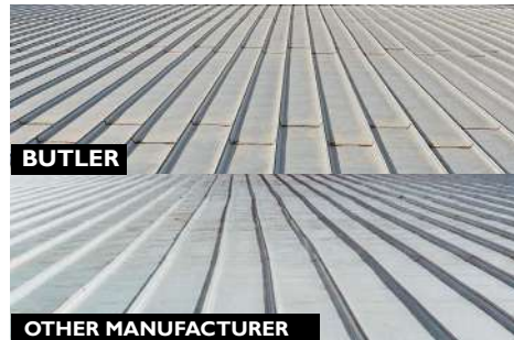
Other Manufacturer Above Top: Butler's factory punching assures straight panel alignment. Above Bottom: Without factory punching, these misaligned panels bind on clips, strain seams and compromise weathertightness.
