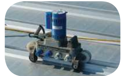
Butler's exclusive Roof Runner® completes the industry's only field-formed 360-degree Pittsburgh double-lock seam.
